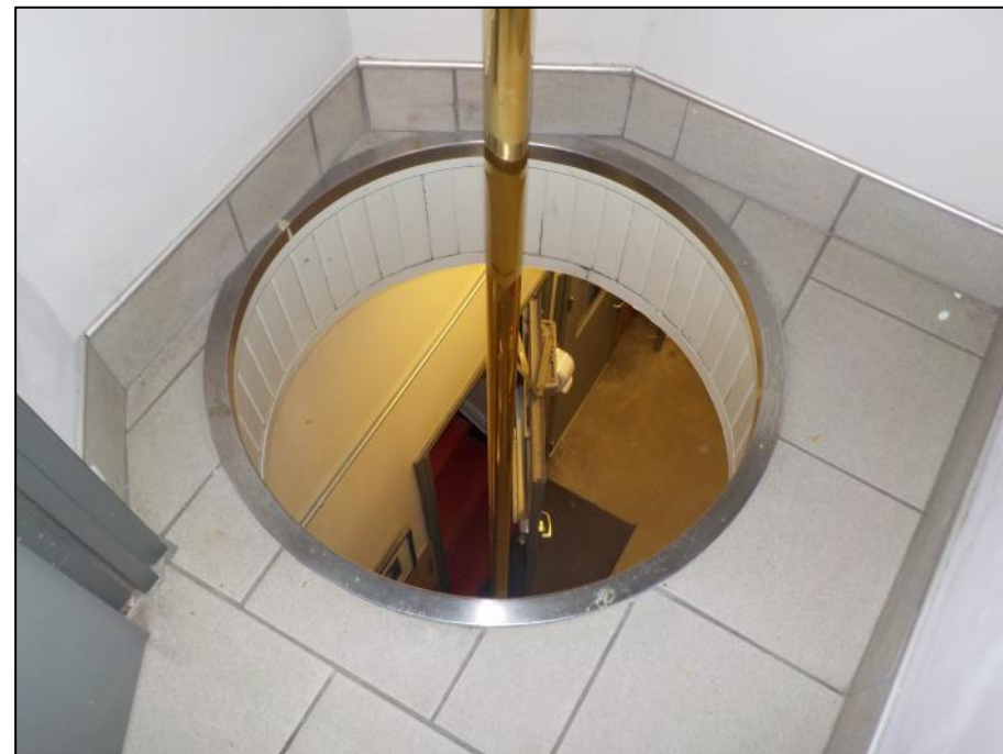
Image 63: Brass sliding pole and chute from second-storey
