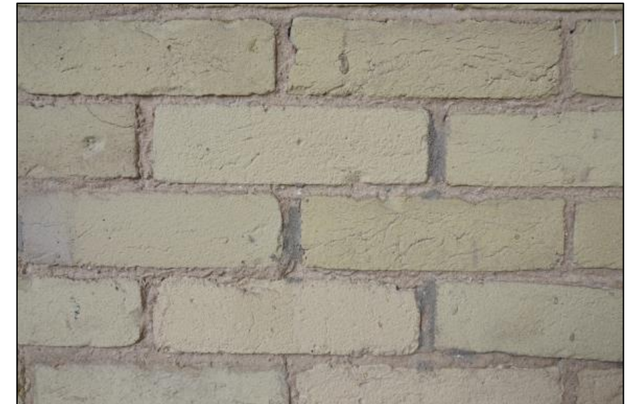
Image 16: Repointing of some mortar joints (east elevation)
