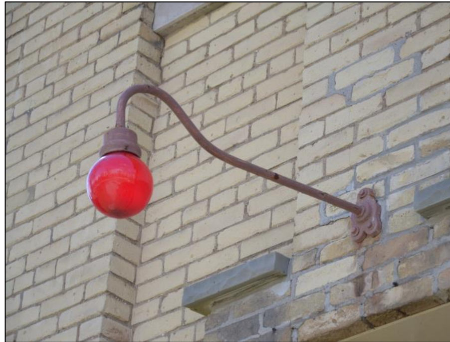
Image 20: East elevation view of period gooseneck exterior lights
