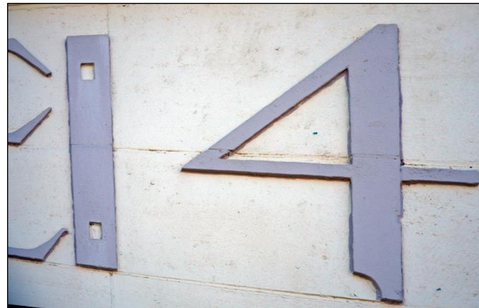
Image 15: Period signage on east elevation- cut concrete lettering
